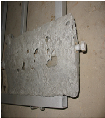
Fig.5: Erosion in the gate
